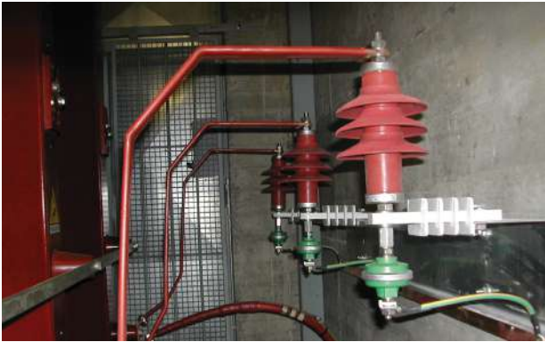
Example of protections for the MV system of the MV/LV transformer with ZU HV 24.2 surge arresters.
