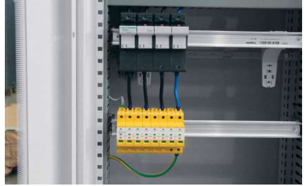
Example of protection with line CB > 160 A.
